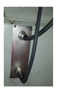
PCE-MWM 240-A VHF-Band Sensor / continuous moisture measurement in bulk (tank / silos)
